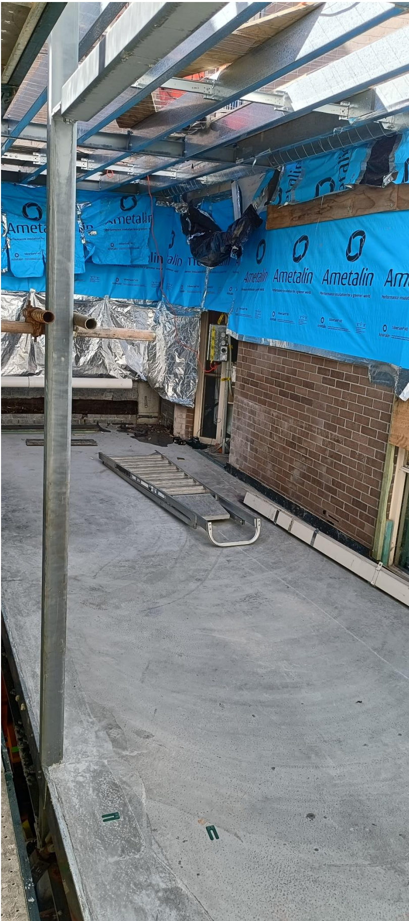
Photograph 16 – ASB connection demolition and adjustments
