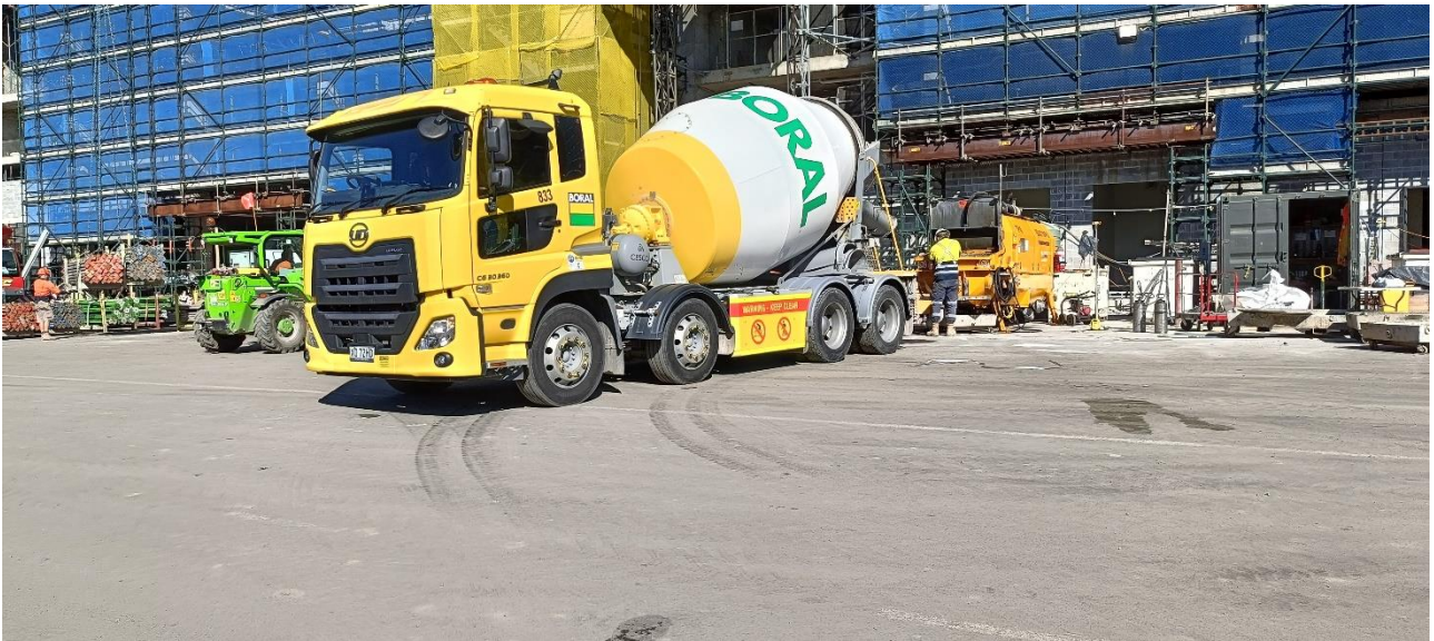
Photograph 13 – Concrete pump setup with spill trays
