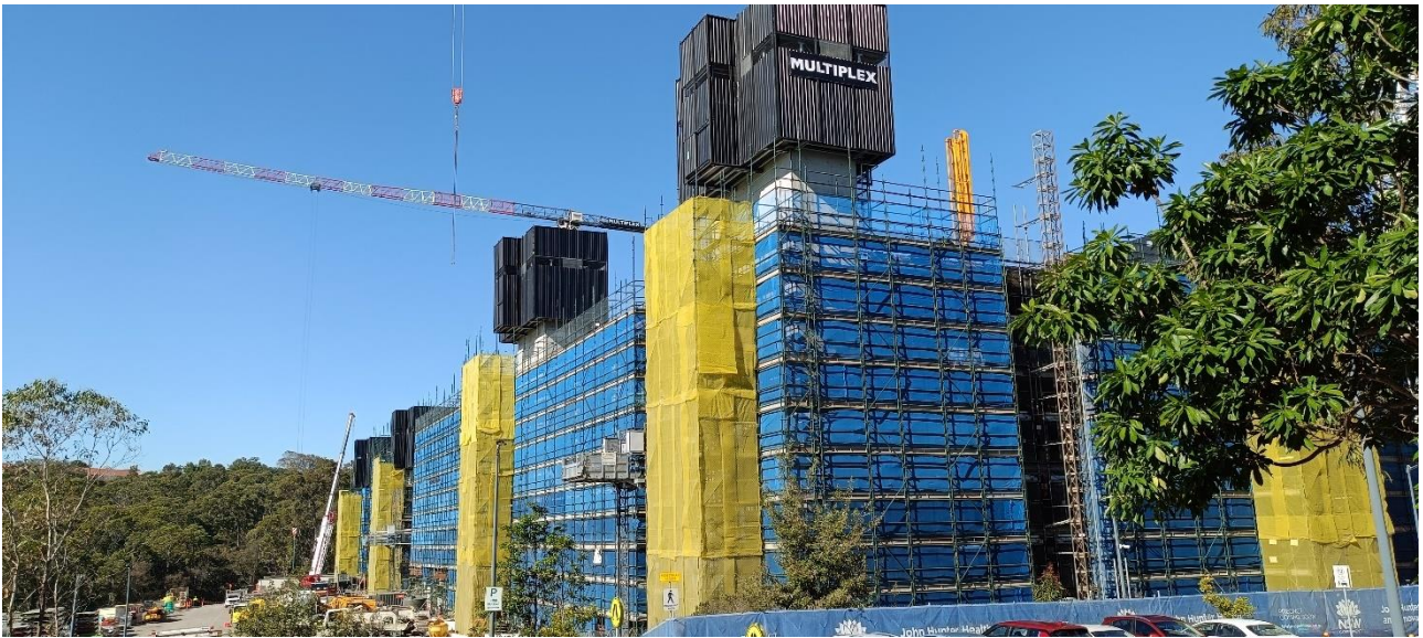
Photograph 5 – ASB looking East
