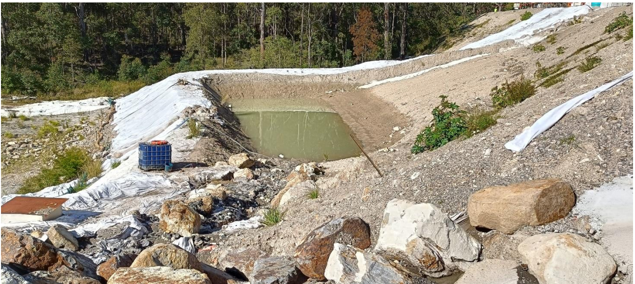
Photograph 12 – ASB sediment basin 1
