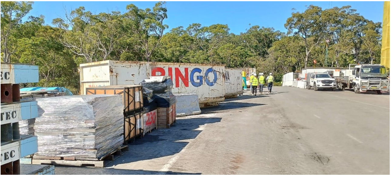
Photograph 15 – Waste bin location
