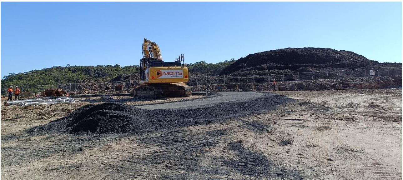
Photograph 8 NICB link roundabout construction
