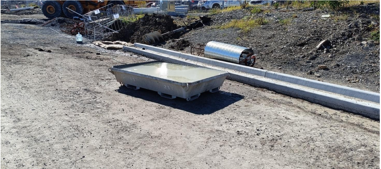
Photograph 7 Concrete washout tray from Kerbing works
